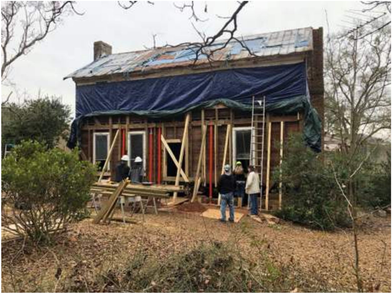
The Lyon Farmhouse, under construction in December 2018.
