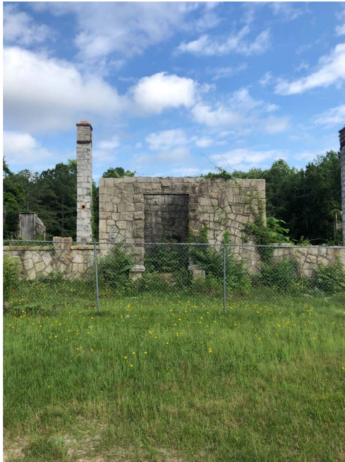
The current status of the Bruce Street School ruins, prior to historic preservation efforts.
