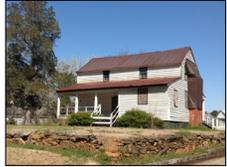
This type of house, Plantation Plain, was common in rural Georgia. The plan features a two story core with a rear shed addition. The room to one side of the front porch is typically called a parson's or traveler's room. Access through a door onto the front porch maintained family privacy.
